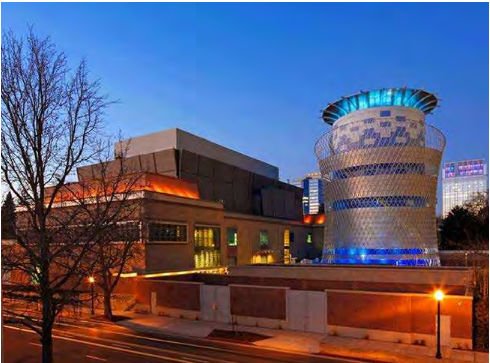
California Dept. of General Services Central Utility
